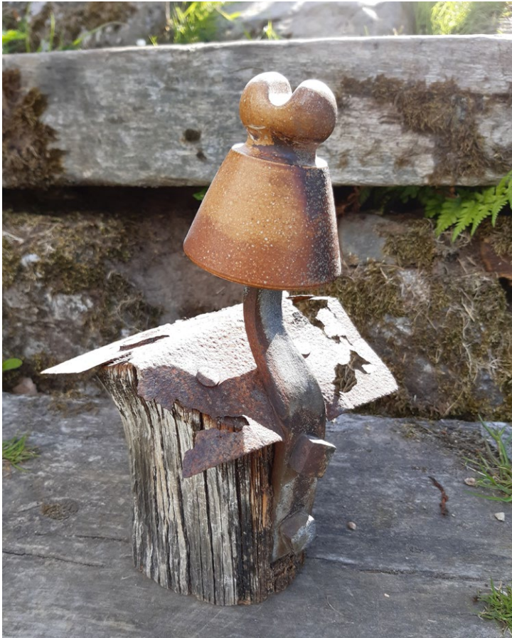
PHOTO 1 – Curtoys Pattern on an original pole top.
