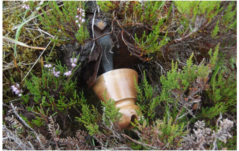
PHOTO 10 – Light coloured Curtoys as found on a fallen pole, hidden in heather.
