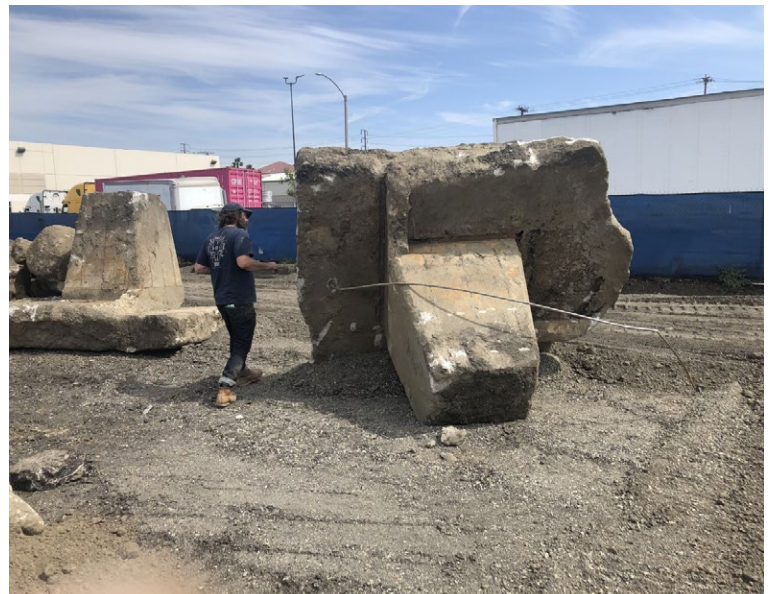
ABOVE: THE LARGE FOUNDATION PIERS REMOVED FROM THE SITE
