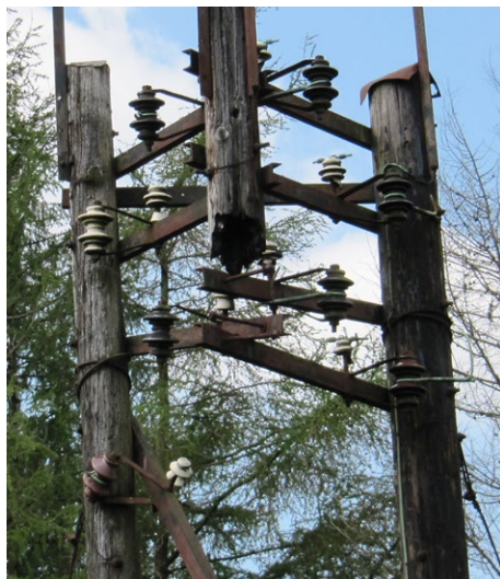
THE BUSINESS END OF THE OLDER 'CORNER POLE' SHOWING THE LARGE SHACKLES
