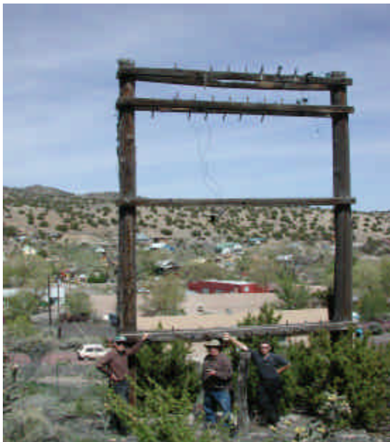
Large Power Frame at Power Plant Site
