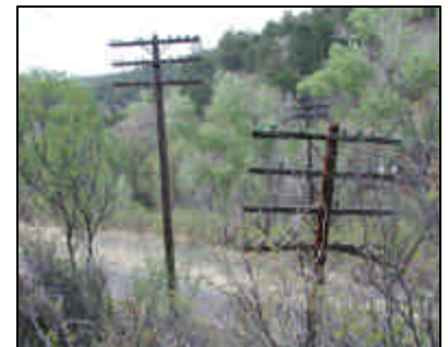
Toll Line Crossing Over the AT&SF Rail Line
