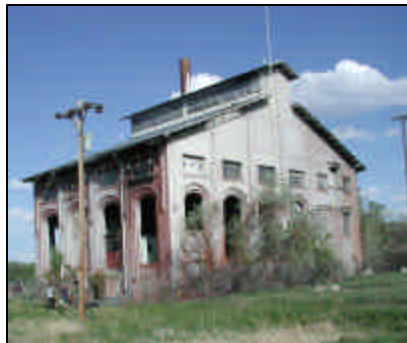
The Old Walsenburg Power House
