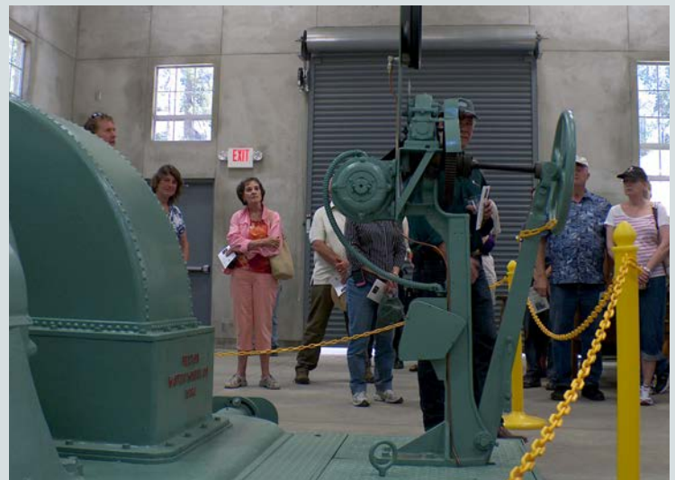
The interior of the powerhouse
