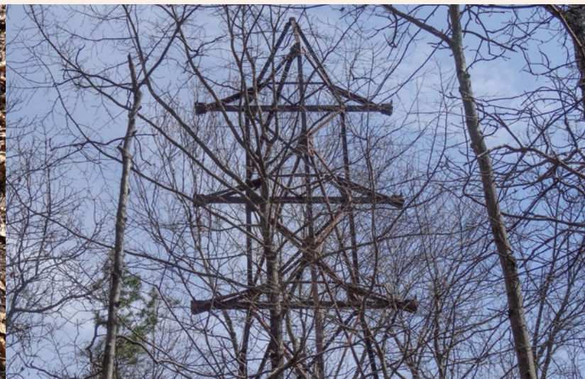
Top of a still standing transmission tower.
