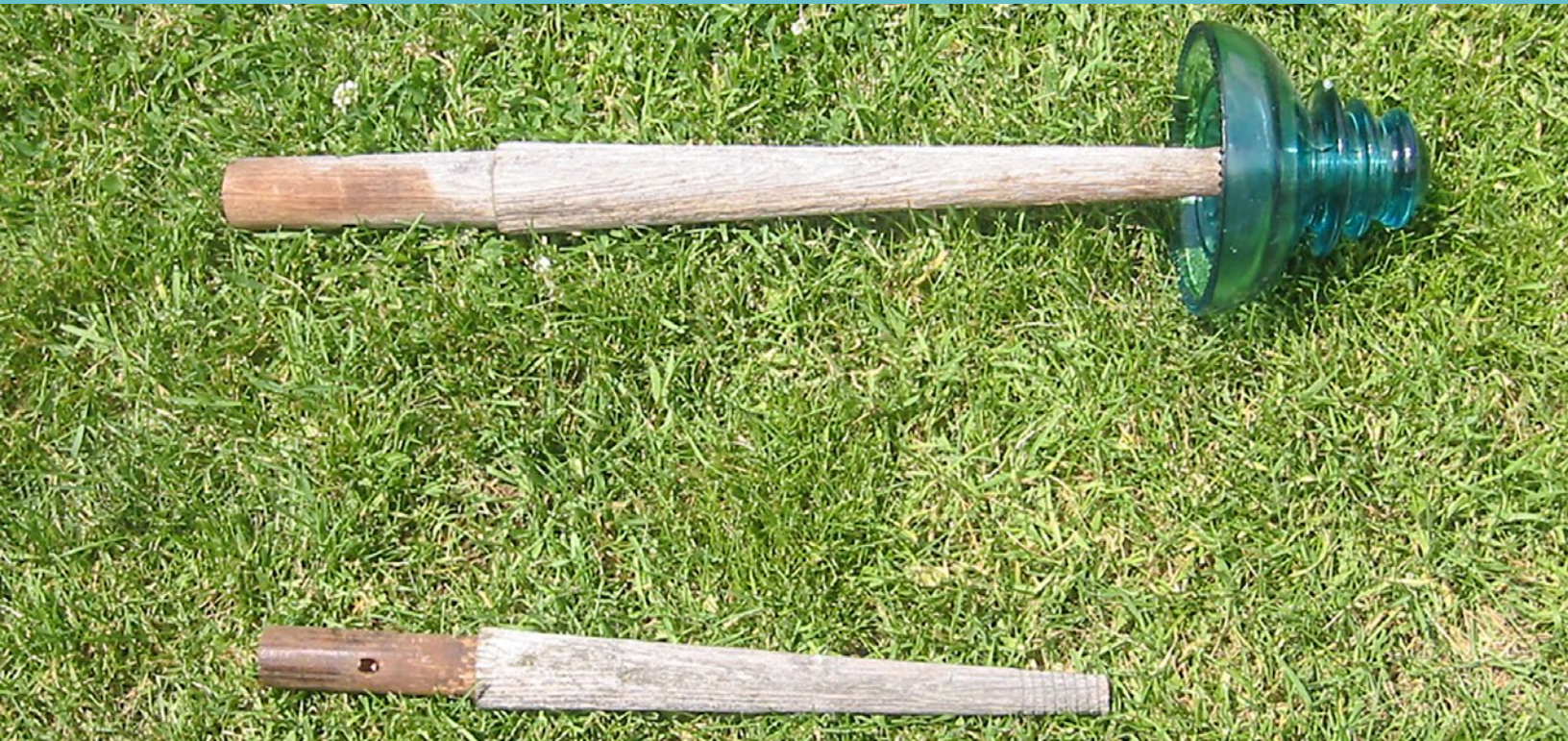
Center Pin 28" and Cross Arm Pin 24" Long
