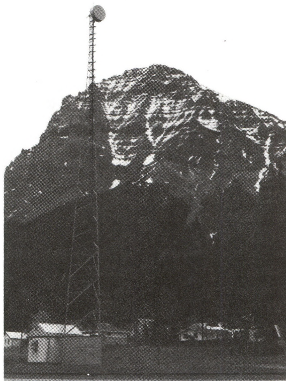
CPR at Field, B.C. Microwave communications have replaced open-wire telegraph lines.
