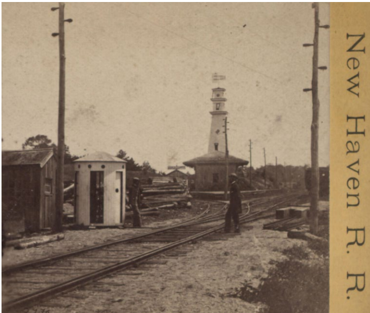
ABOVE: THIS IS AN 1860S PHOTO OF HOOKS IN USE ON DRUMSTICK ARMS AT A NEW HAVEN, CT RAIL YARD. THIS IS THE SAME TYPE OF CROSS ARM USED ON THE SHANK TYPE HOOKS WHICH HAD HOLES FOR TIE WIRES IN LIEU OF HOOKS
