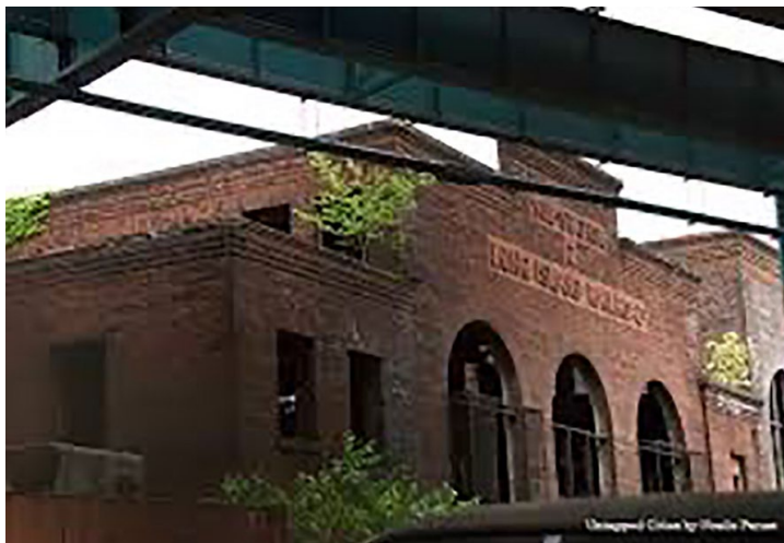
SUBSTATION ABANDONED, MODERN ERA
