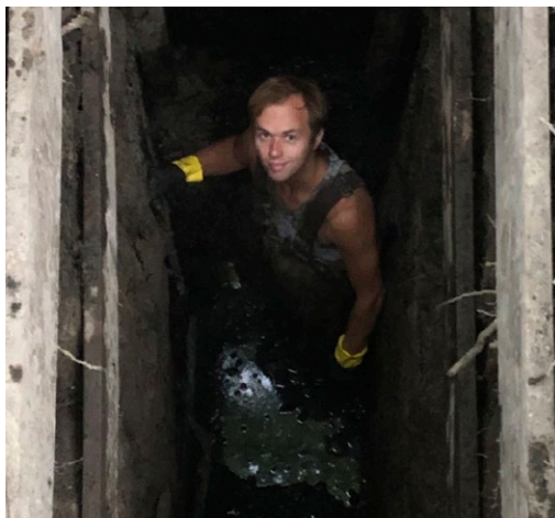
I DUG THOSE BY HAND WITH THE HELP OF A FRIEND BUCKETING OUT MUD. WE HAD TO BRACE UP THE SIDE TO PREVENT COLLAPSING AFTER ABOUT THE 9' MARK. THOUGH THE INSULATORS WEREN'T FOUND IN THOSE PITS, SOME UNBELIEVABLE FINDS WERE DISCOVERED.
