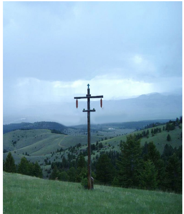
MY RENDITION OF A COCHRANE POLE HEADING TO VIRGINIA CITY FROM THE SWITCH STRUCTURE
