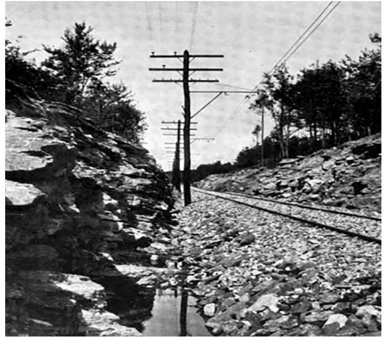
Hammerrock Pass, located in Charlton, showing the pole construction typical to the railway line.
