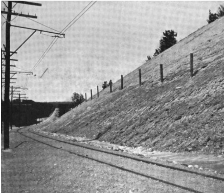
Deep Cut was where the cars hit more cows and other animals, so the railway installed fences to prevent delays and deaths.
