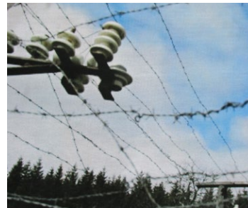
ABOVE: CERAMIC INSULATORS ON ORIGINAL ELECTROZAUN
