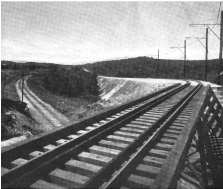
One of the many well-engineered timber bridges on the railway. Here is the crossing over Webster section of the Boston & Albany railroad. The Boston & Albany Railroad opened in the mid 1840s.
