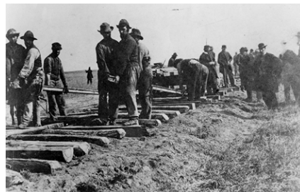
UPRR CONSTRUCTION CREW
