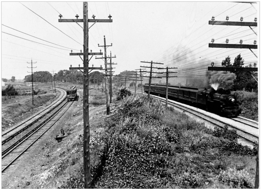
A Chicago, Aurora & Elgin interurban on the left, Chicago & Northwestern Freight train on the right. M-2332 multipart insulators plainly visible on the pole line.
