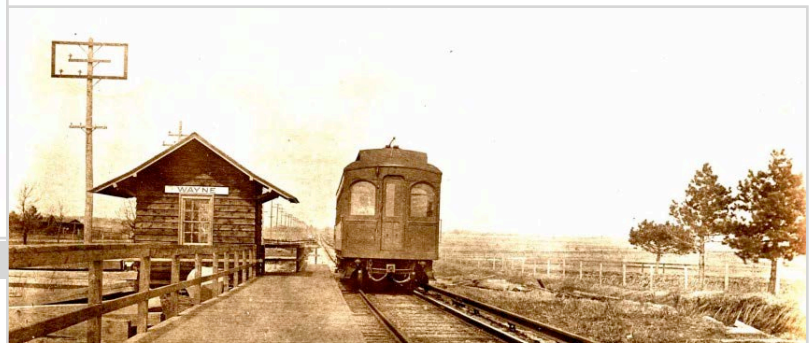
Train Station at Wayne, IL showing unusual frames around insulators
