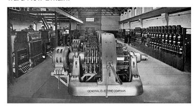
Interior of Waterbury Substation No. 1 Showing Transformers, Rotary Converters and Switchboard. (\*5)
