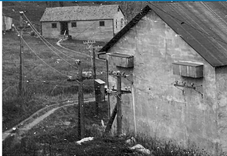
33,000-volt Circuits Exiting the Powerhouse Through "Pigeon-Coops". (Unknown photographer)
