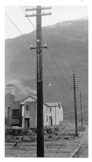
**Photo 1** – A view of some poles in Kinlochleven between 1905 and 1909, showing cable insulators for lighting and telephone lines higher up.
