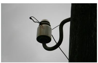
**Photos 14&15 (Above)** – G&G cordeaux on a fallen pole & A Bullers trademark piece on a swan neck bracket.
