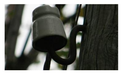
**Photo 13** – A bright white (European made) slot top, probably used to carry the same wire/cable as the small tapered insulators seen further down.
