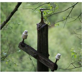
**Photos 7&8** – Large India pattern slot top insulator in situ & the top section of the same pole with one surviving cordeaux.
