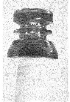
l to r: 3 3/8" h (dark aqua) embossed F: GAYNOR; B: NO. 6--3 1/2" h (dark aqua) embossed F: GAYNOR; B: NO. 91--this 1 7/8" h (aqua) no name, hole thru was used on the old 14 twisted pair telephone lines, and was taken off a house by Elmer in 1918. It was attached using a 3/8" lag screw.
